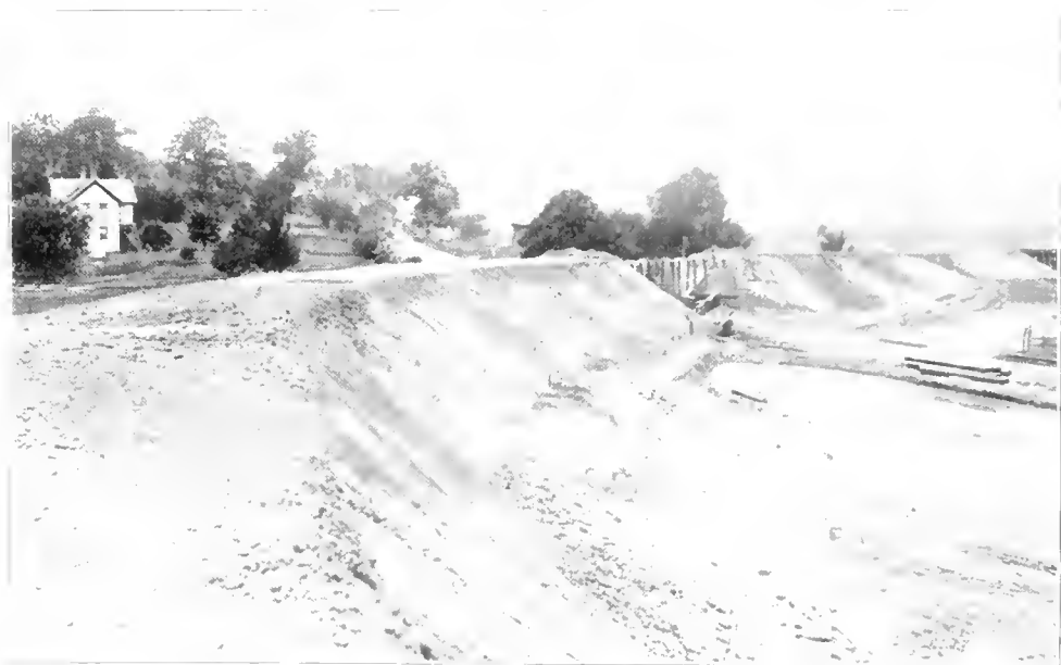
SCENES ON THE NEW RAILROAD GRADE
